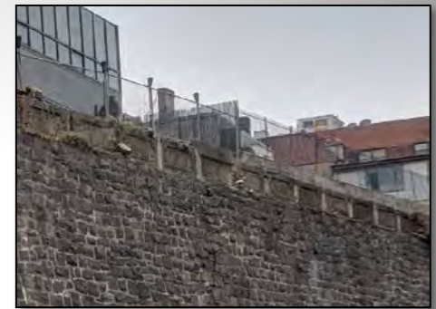
Existing Parapet top of the Wall
