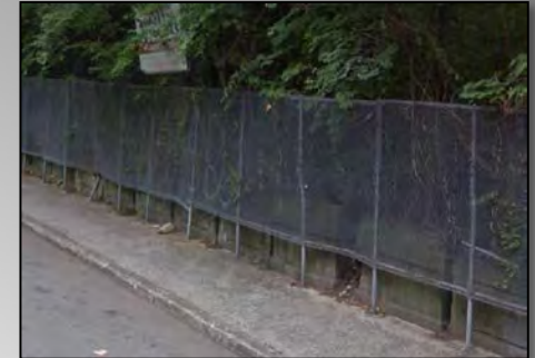
Existing Parapet on the East side of the roadway
